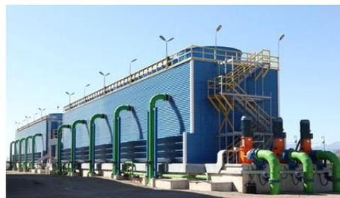
**Figure 7. Cooling Tower Battery**
