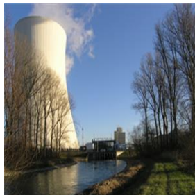
Figure 4. Commercial Cooling Tower
