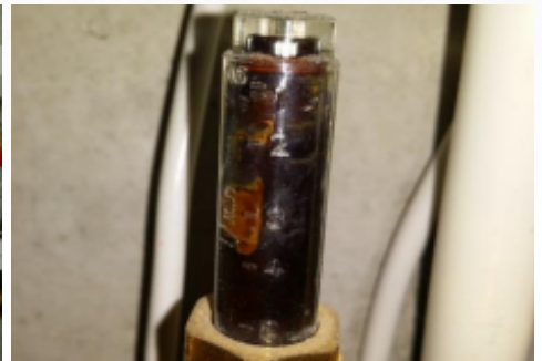
Figure 3. Closer look at the brown, slimy deposits caused by bacteria
